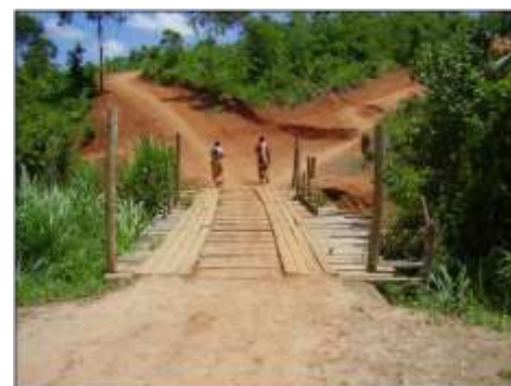
Bridge built by GRL, Idete Village, Tanzania demand is very high and we expect to sell all production in Tanzania, with some possible added export to Kenya.
